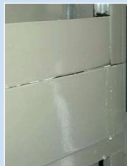
Jalousies alu Infiltration interface traverse/montant.
