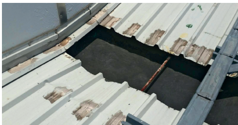
Photo : © SARETEC - Pierre LAMORIL
