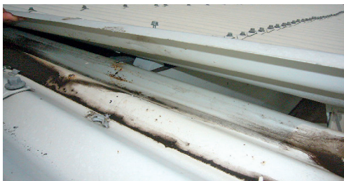
Photo : © SARETEC - Pierre LAMORIL
